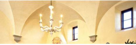
Unlike marble it has a single, soft color with subtle shadings. It is a natural material made of lime and ground marble.
